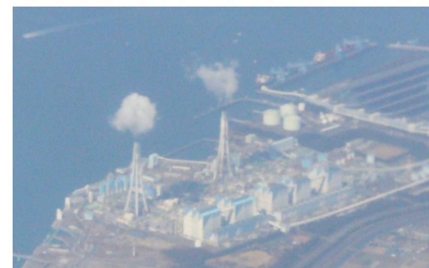
Hekinan power plant
