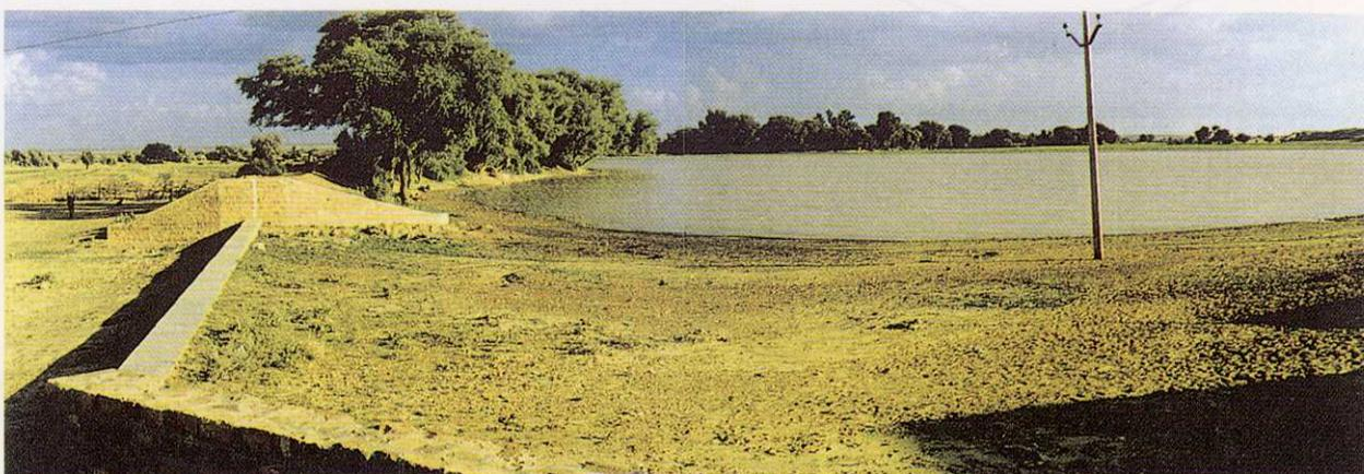
**Fig. 8** Khadin - A traditional rainwater harvesting system for crop production.
