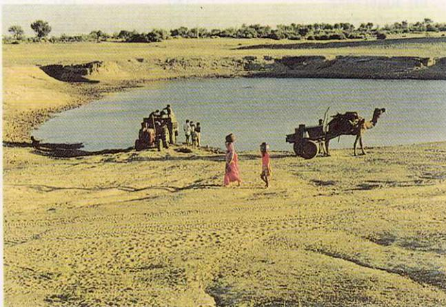
**Fig. 7** Nadi (Village tank) - A traditional rainwater harvesting system for domestic water supply and livestock consumption.
