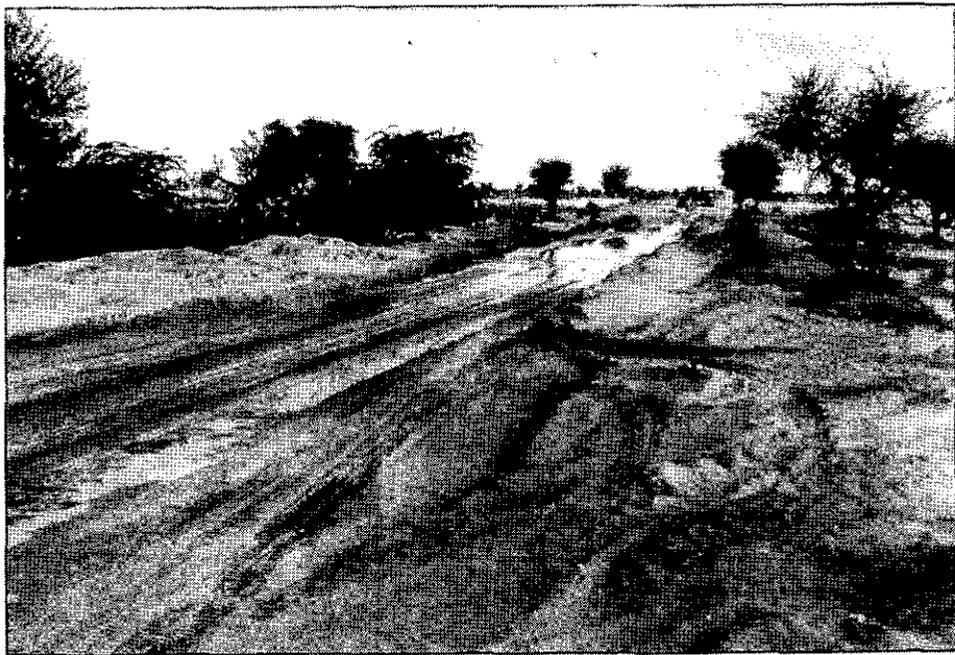
Fig. 2.15 Sand pile on Tinwari Osian Road (Jodhpur, India) becoming muddy during rain and disrupting vehicle movement.
