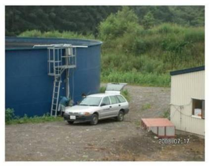
Storage Tank: 23m diameter / 4.5m depth Store 150 heads of milking cow slurry around 180 days 20kg of CH<sub>4</sub> & a few N<sub>2</sub>O emit./day
