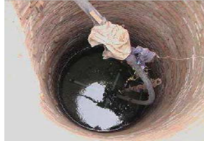
Lowering ground water table
